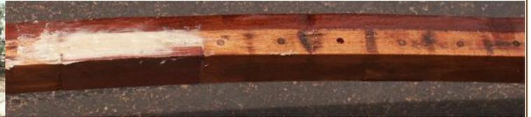
Shown above is one of the main arch beams reconstructed and sistered to new material to provide additional strength. This actually increased the width of the beams by 3/4" which was necessary to ensure structural integrity was regained.
